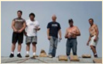
Volunteers in Action Roofing the Office
